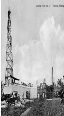
Circa 1922, Oil well installation near Oldsmar, Florida in Pinellas County.
